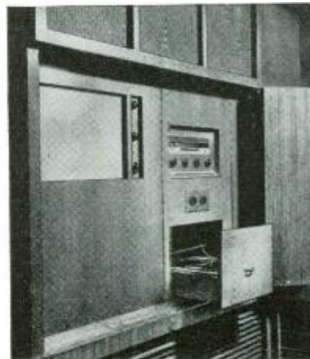
Fig. 5—Closed doors hide this installation.
